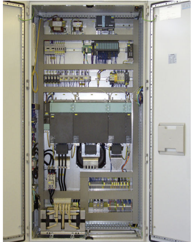
Control cabinet with SINAMICS S120 in bookshelf format
