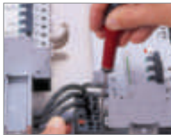
Prefabricated connections, optimised and fully insulated.
