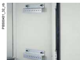
Perforated Rails Installed on Lateral Studs.
