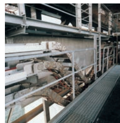
310 plastic chains and 45 stainless steel chains applied to "Oresund Bridge" between Sweden and Denmark.
