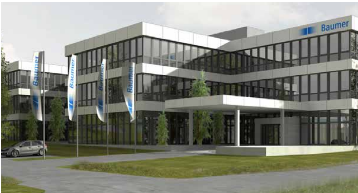
High-Tech Center Bodensee with distribution center and head office of Bourdon-Haenni GmbH
